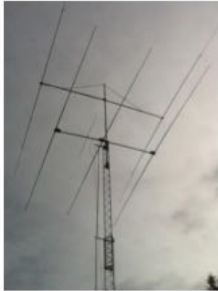
Normal station antenna
